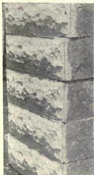
FIG. 65—COMMON VARIETY OF WHITE ROCK-FACE BLOCK
